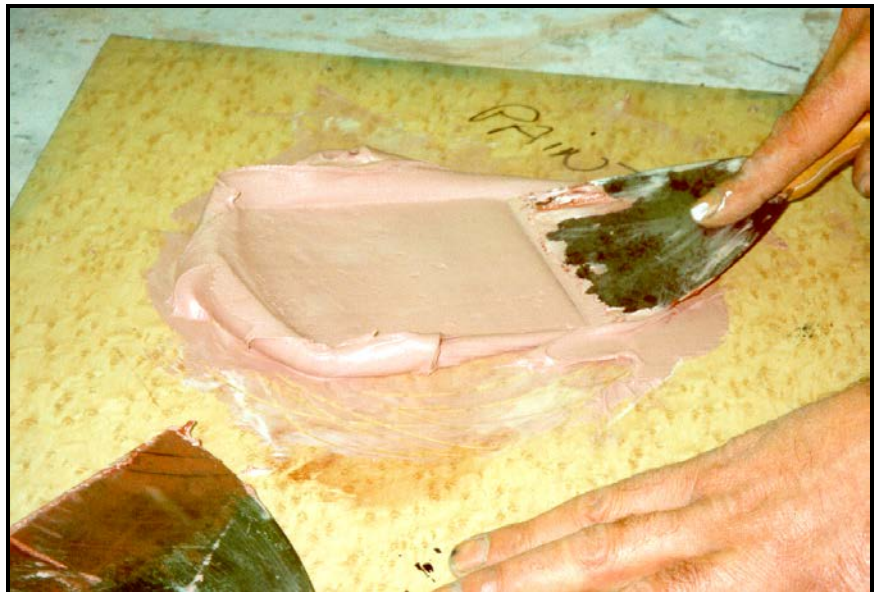
Fig 24. Epoxy fillers must be mixed thoroughly to ensure complete incorporation of the two components. Protective gloves should always be worn whenever mixing or applying epoxy materials!
